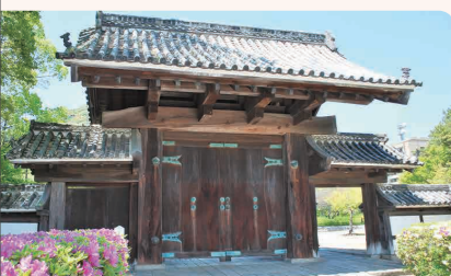
↑ Former Yamaguchi Clan Office Gate The important cultural asset of Yamaguchi Prefecture.
